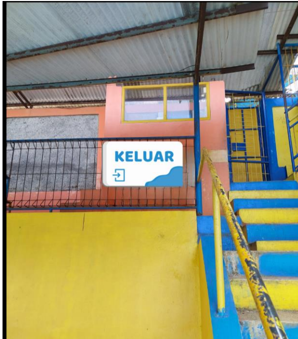
Gambar 16. Implementasi Directional signage
